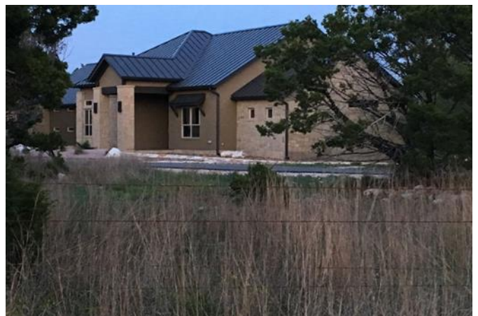
Our fence line to our front porch 151'
