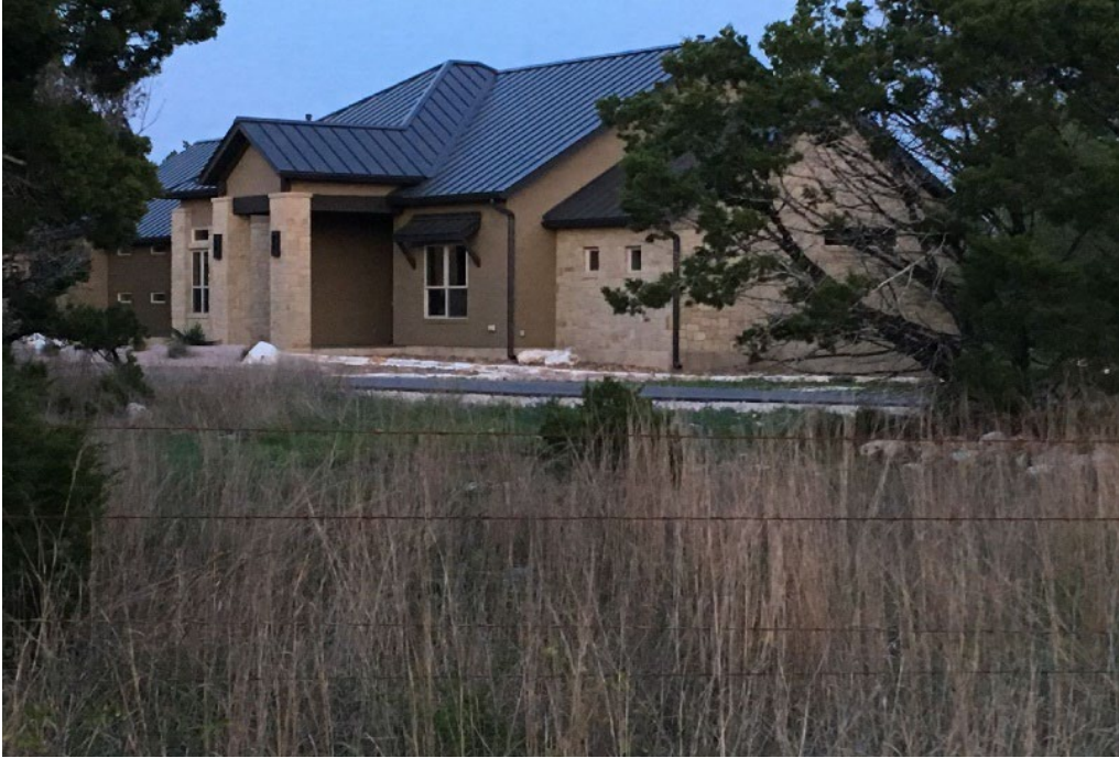
Figure 2, showing Ms. Guckian's fence line (foreground) 151 feet from her fence line. 3
